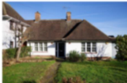
(above) Some of the bungalows at each end of the two-storey brick houses have flat windows instead of the bay windows used on type A81.
